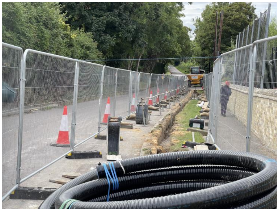
Work on the Heating Scheme in progress by the school, The clunch has been a difficulty, as so too the (very) old electricity power cables, which are brittle and very near the surface. Photo by Peter Rand.
