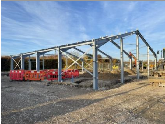
Erection of the steel framework for the energy centre up on the Heath...
