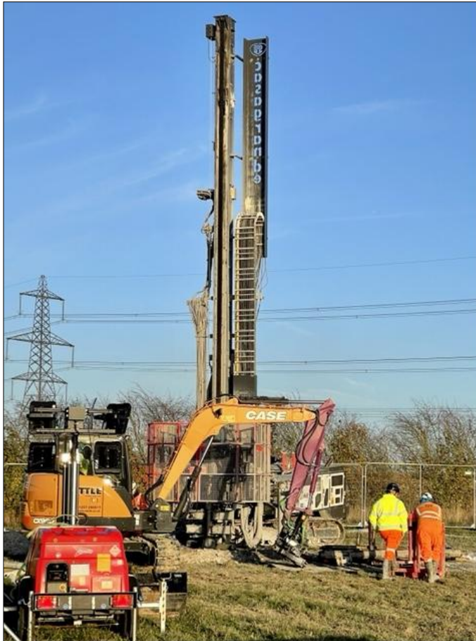
The huge drills making the bore holes for the heat extraction up on the Heath
