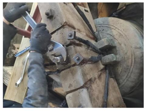
It's all happening - here's a picture of the last nut being unscrewed so the headstock can be taken away for rebuilding.
