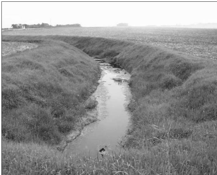
Drainage ditch, cut only on the top with margin on top of bank
